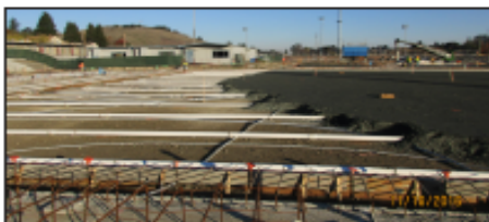
Gymnasium Piping and Drainrock
