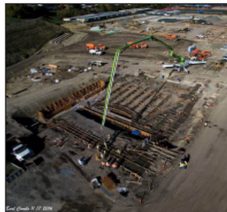
Concrete pour, Performing Arts building
